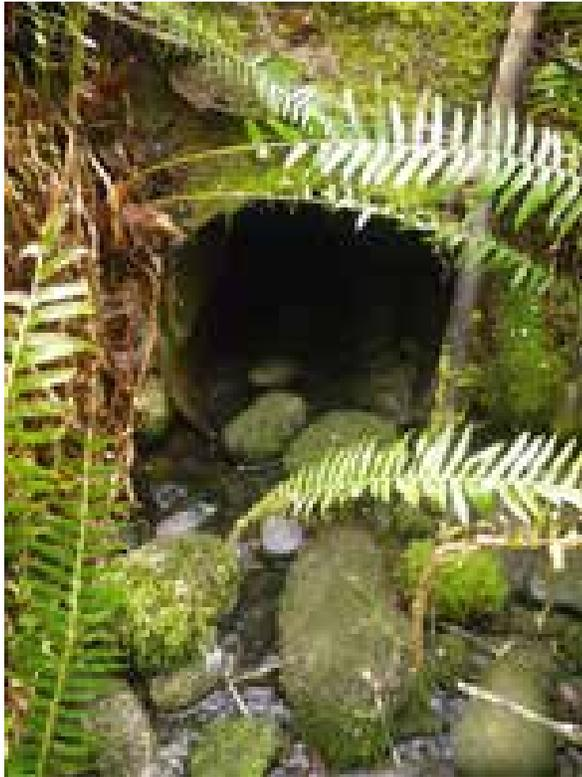
Outflow of the subject watercourse on the northern side of the Cowichan Valley Trail. This existing crossing would remain in place, but an overflow culvert would be placed through the trail at a higher elevation than the existing culvert to serve as an overflow when the stormwater retention area is at maximum capacity.
